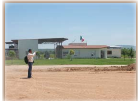
office and storage shed
