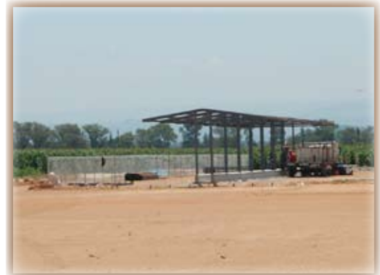
pens and shelters under construction
