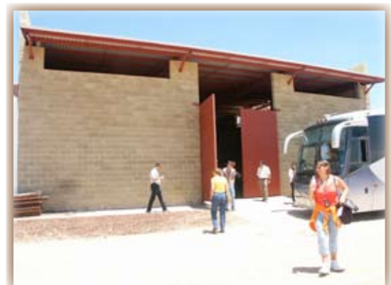
exterior of the hay shed
