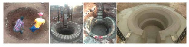
The runway needs to run all the way to the bottom of the pool so that goats can easily walk out of the pool. The whole dip needs to be fenced off so as to restrain the goats while they are waiting to be dipped. The runway needs to be fenced and have a gate at the end for goats to be released once they have dried. The farmers need to stand between the runway and the pool to submerge the goats with a cleft stick and also use the cleft stick to assist goats out of the pool.
